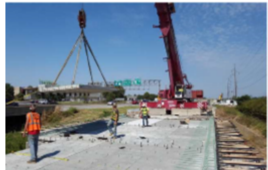
Placement of 25-foot precast deck panels.
