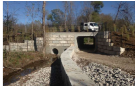
A large block wall diverts low-flow events into double 48-inch reinforced concrete pipes.
